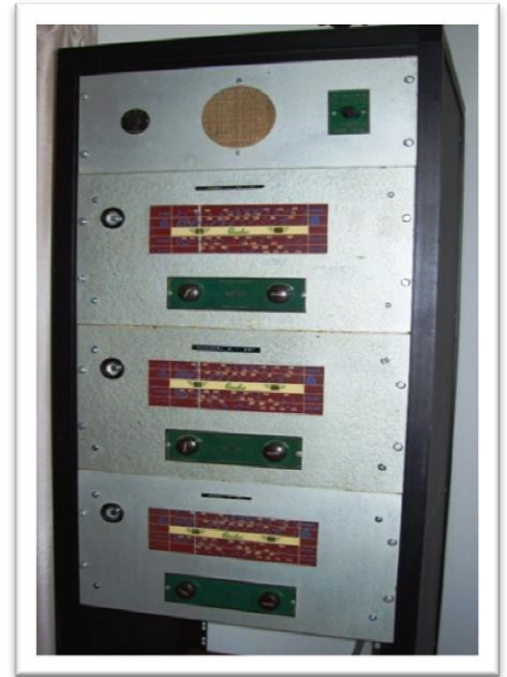
Audio Engineers Hospital system that was originally installed in the Shoalhaven District Memorial Hospital NSW, installed in 1952
